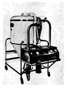
Portable spray dryer unit for pilot and small scale production. Unit is constructed of stainless steel, with two built-in heaters, one electric and the other direct fired gas, both controlled directly from the panel control board **PE8**
